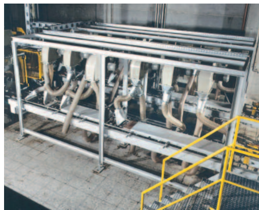
RTR drying line and RQS quality check before packaging
